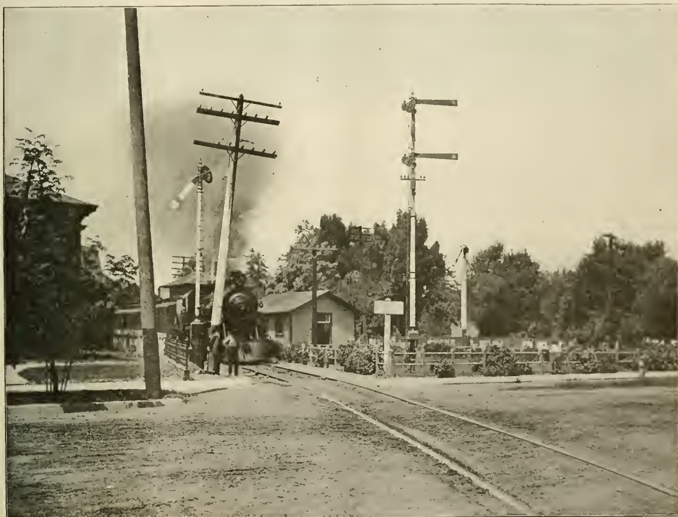
ON THE LINE OF THE SOUTHERN PACIFIC RAILWAY, SAN JOSE, CAL.
